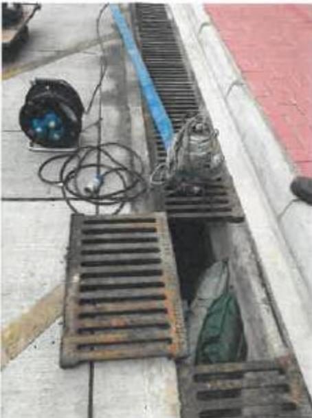
Figure.3 Sandbags were placed at the nearby storm water channel
